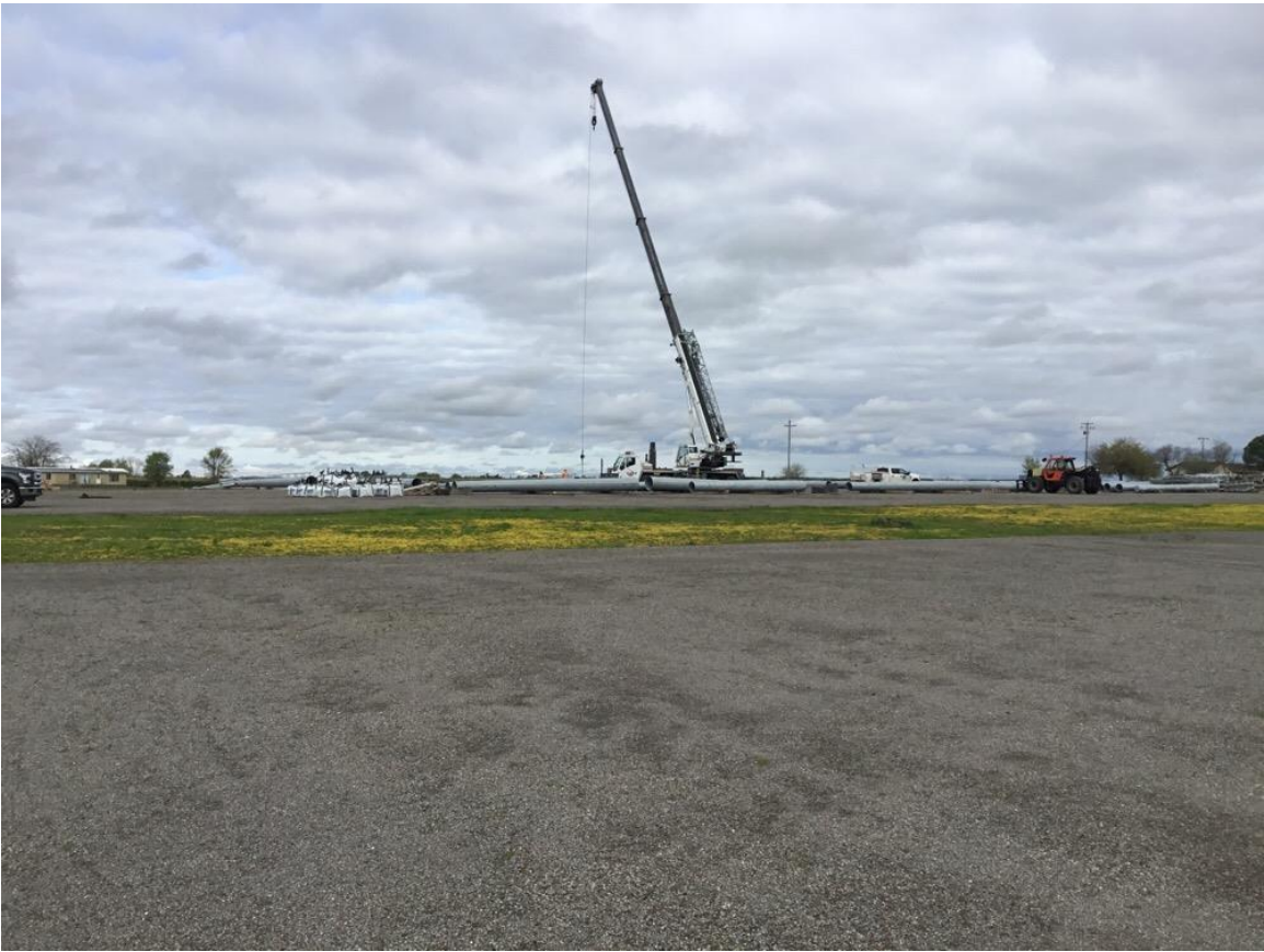
Photo 1: Crews working to assemble new poles at Landing Zone (LZ) 9/67.
