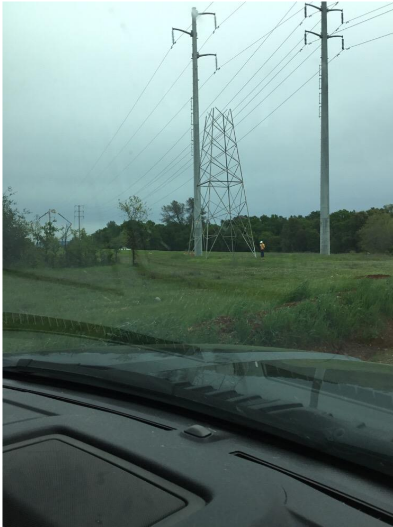
Photo 2: Tower removal in progress at location 1/12.
