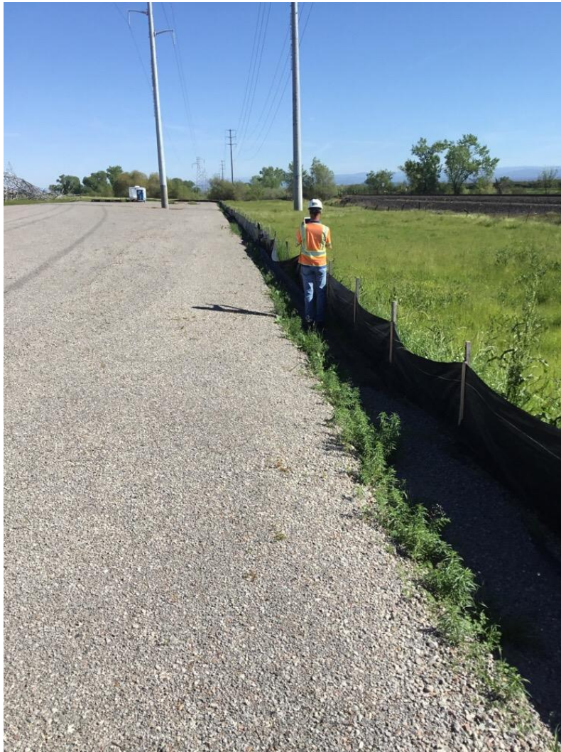
Photo 3: Maintenance of silt fencing SWPPP BMPs observed near LZ 9/67.
